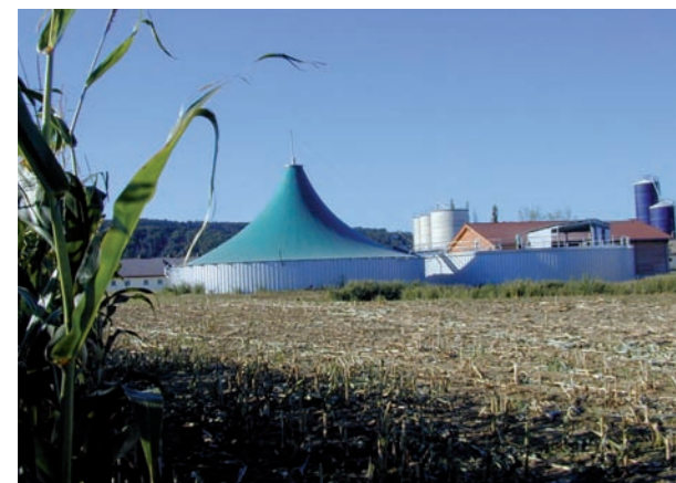
Photo 11: General view of a 2-step crop digestion plant with digester 1 (right) and combined gas collector and digester 2 (left)
