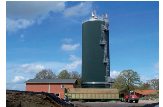
Photo 15: Dry continuous digestion
