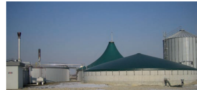
Photo 14 : General view of a 1 MW e crop co-digestion plant using two parallel digesters (left background) and a covered final digesterate storage tank (centre foreground). Gas storage is integrated in digester 2 (background) and in the final storage tank (foreground), further storage capacity is provided in a dry gas storage tank (background right).
