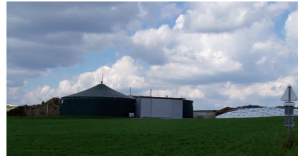
Photo 12: General view of a 2-step crop digestion plant with digester 1 and digester 2 combined with membrane gas collector. The silage clamp can be seen on the right.
