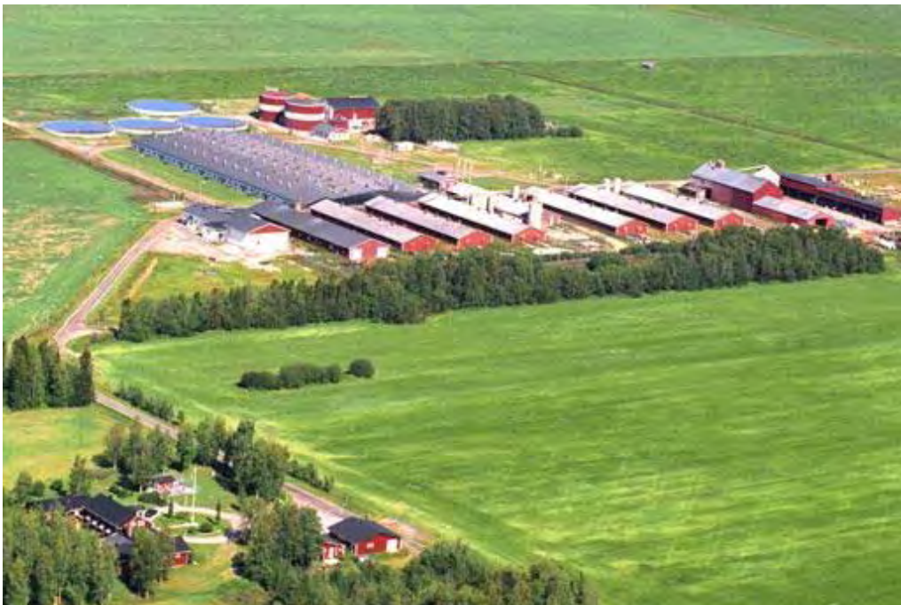
Figure 4.8.1 Photograph of the biogas plant in Alvik
