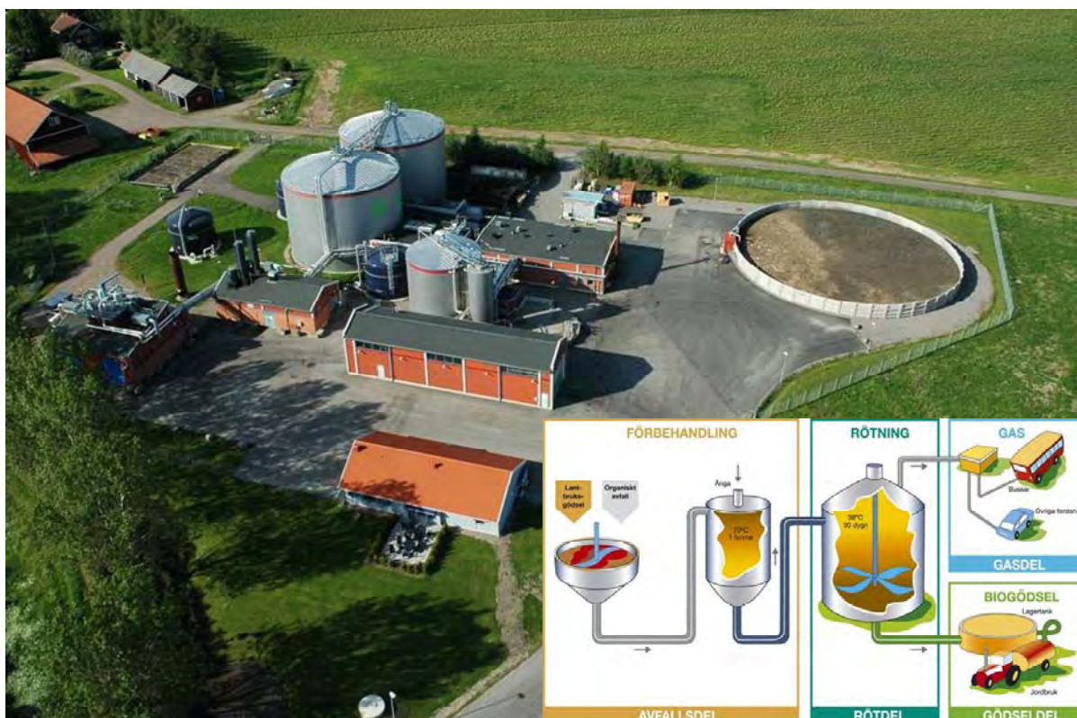
Figure 4.4.2 Aerial photograph of the biogas plant in Linköping, with a schematic diagram of the plant
