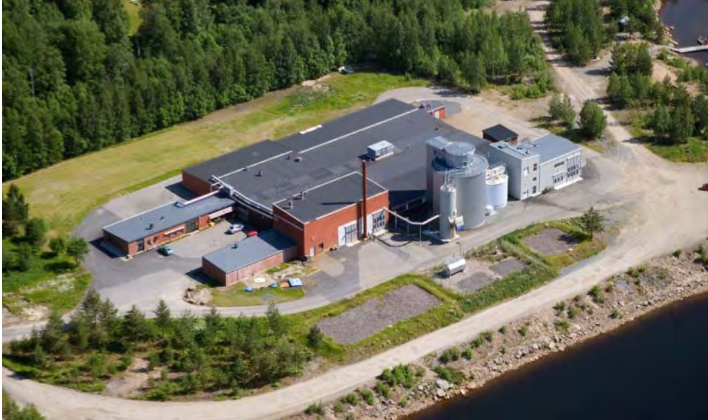
Figure 4.1.1 The biogas plant at Svedjan, Boden
