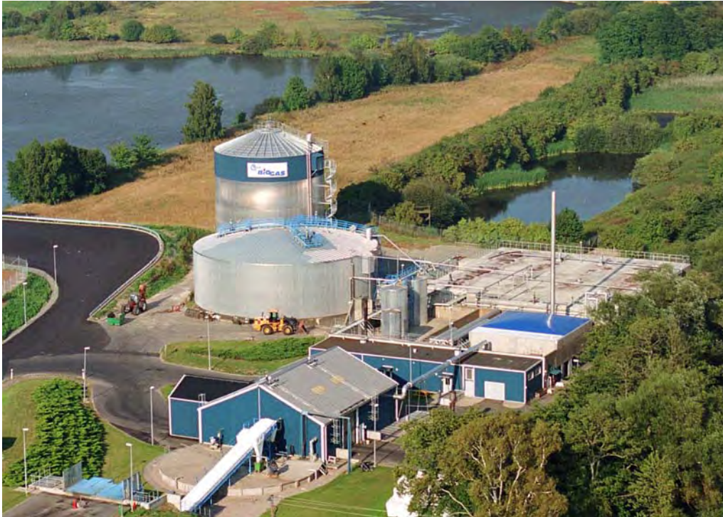
Figure 4.3.1 The biogas plant at Karpalund, Kristianstad
