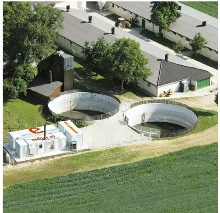
Austria's first biogas feeding-plant injects purified biogas into the existing gas grid.
