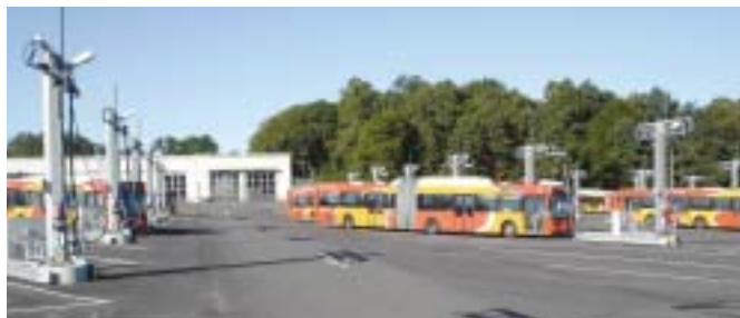
Slow filling system for city buses in Linköping Photo: Svensk Biogas
