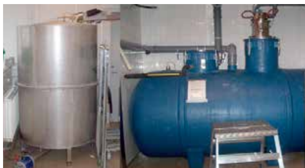
Figure 13: Two examples of throw-ins for large grinding systems (Source: Stockholm stad)
