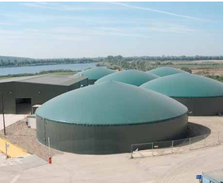
Figure 5: The Cassington AD facility in Oxfordshire, United Kingdom. The biogas plant processes source separated municipal and commercial food waste (Source: www.biogas.org.uk )
