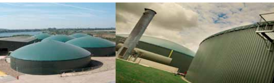
Figure 39: Agrivert Cassington Anaerobic Digestion Plant
