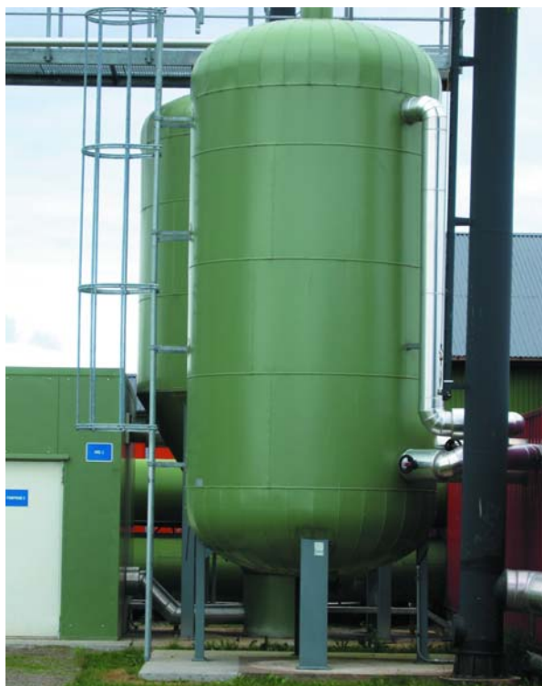
All raw material to the digesters is pasteurised in two batch type pasteurisation units
