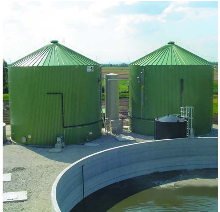
Fig.1: Overall view at the two digesters of the biogas plant Marchfeld. Between the digesters the desulphurisation reactor is situated.
