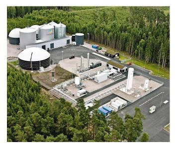
**Figure 1:** Aerial view of Lidköping Biogas plant. The digesters can be seen in the top left corner of the picture, with the water scrubber for biogas upgrading adjacent. Next to that is the liquefaction plant and at the front of the site is the refuelling station (bottom right of picture). Photo: Gothenburg Energy
