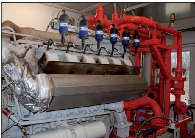
Figure 5: The 360 kW motor-generator (Photo: Michael Tersbøl, Organic Denmark)
