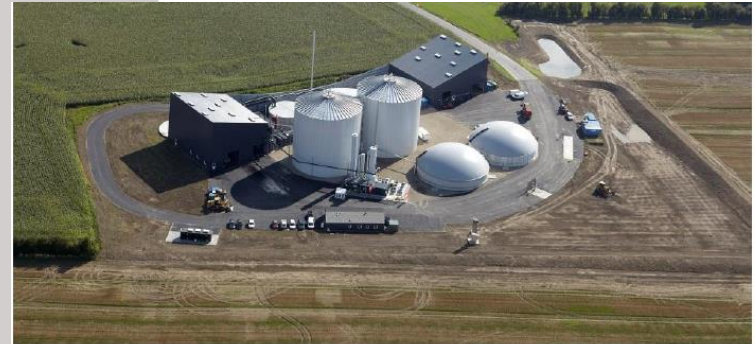
Bio-natural gas plant at Horsens Biogas connected to DONG Energy's gas distribution network in East Jutland. The upgrading facility is the container with the three columns in the centre of the photo. Commissioned in October 2014. Photo: Jørgen Weber.
